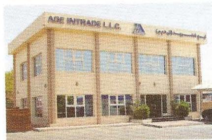
Age Intrade's office building ... over the years, the group has become one of the major players in the local steel market
